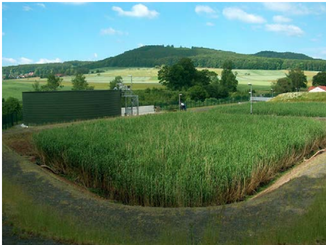
An example of a constructed reed bed – proposed for Burgoyne Bay regarding treatment of liquid waste
