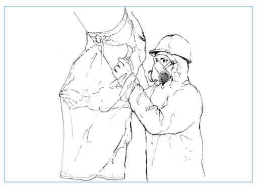
When using glove bags, follow the manufacturer's instructions and wear appropriate PPE (at a minimum, this should include disposable coveralls and a half-face respirator equipped with P100 [HEPA] cartridges).
